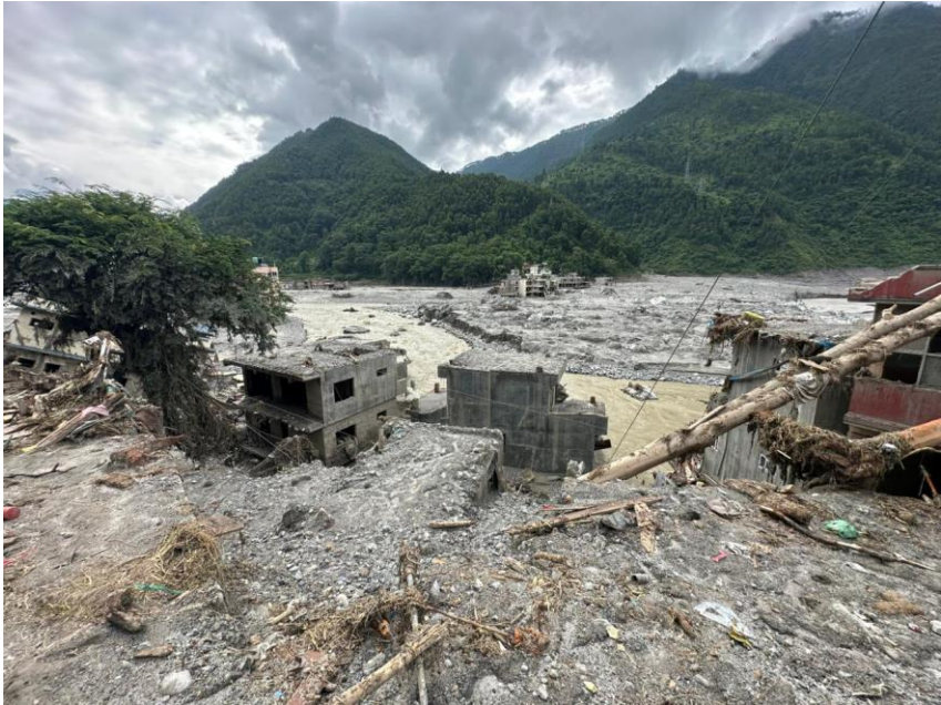
A view at flood-impacted area of the Betrawati Bazzar (Photo Credit: Saroj Adhikari)
