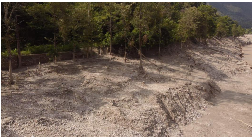
Figure 13: A section of river bank impacted by the floods
